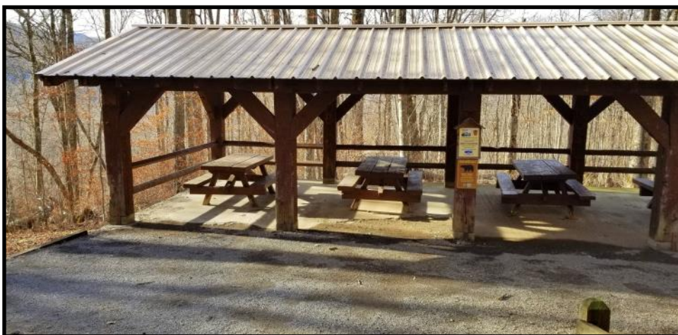
Left: New metal roof on the picnic shelter
